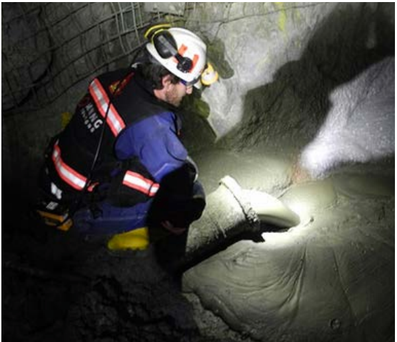
Underground Backfill. Photo: Sika Canada
